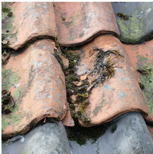
dak [2]-west: gebroken pan
